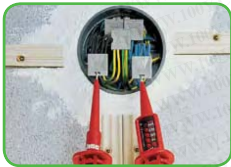
Voltage testing of push-wire connectors
