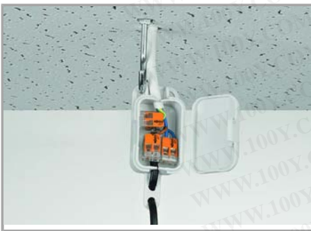
Pendant light connection in suspended ceilings
