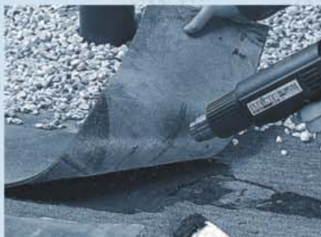
Welding roofing felt
